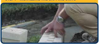
The job is almost done! Using a suitable landscape grade outdoor adhesive (such as landscape liquid nails) place 4 'blobs' of adhesive on the top of each block on your top course. Once you have done this, firmly place the capping unit into place on top of the glue.
