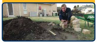
You can continue laying blocks by simply stacking them on top of one another — just like using children's blocks! Make sure you have a small hand broom to sweep dirt and debris off the top of the course below to ensure your laying blocks on a nice flat surface.
