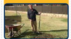
Remove the turf and debris from the area to avoid them growing back through your veggie patch! Then around the shape of your veggie patch which has been marked out, excavate a trench approximately 50-100mm wider than the block and approximately 200mm in depth.
